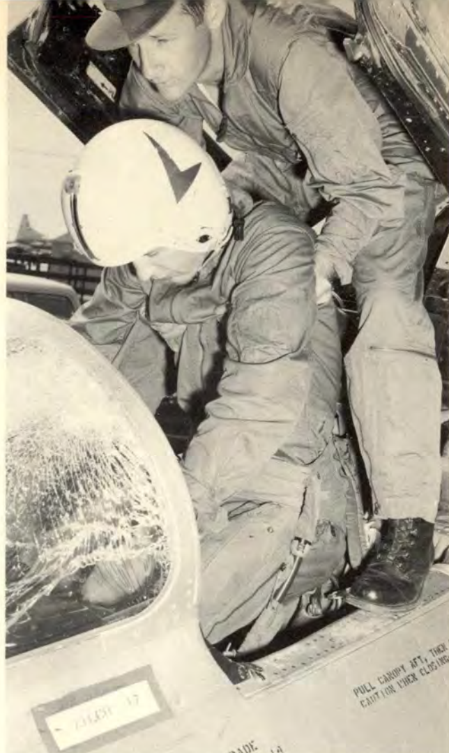
for rescuer to stand on rails behind seat, pull pilot's feet into the stirrups and lift him from seat.
